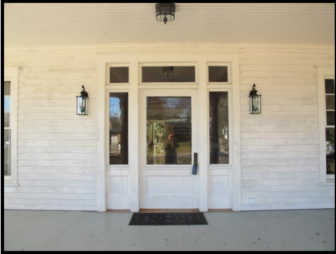
Figure 2.2-3: View of Ranson House (MK1351), Main Entrance Looking West.
