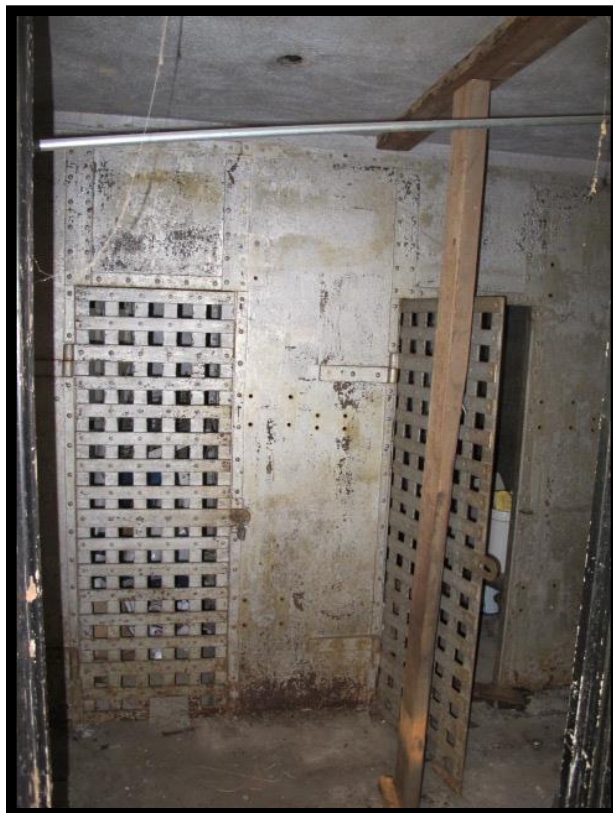
Figure 2.2-36: Huntersville Town Jail (MK3299), View of Cell Block Looking North.
