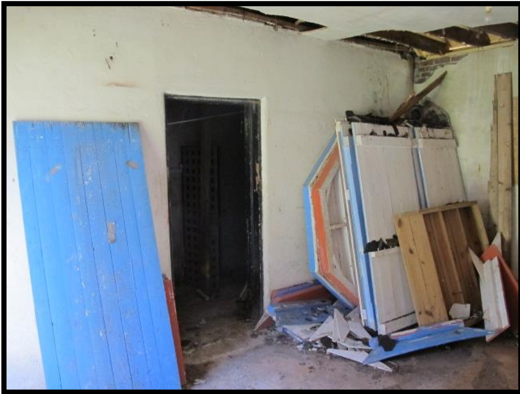
Figure 2.2-35: Huntersville Town Jail (MK3299), Office Space Looking Northeast.
