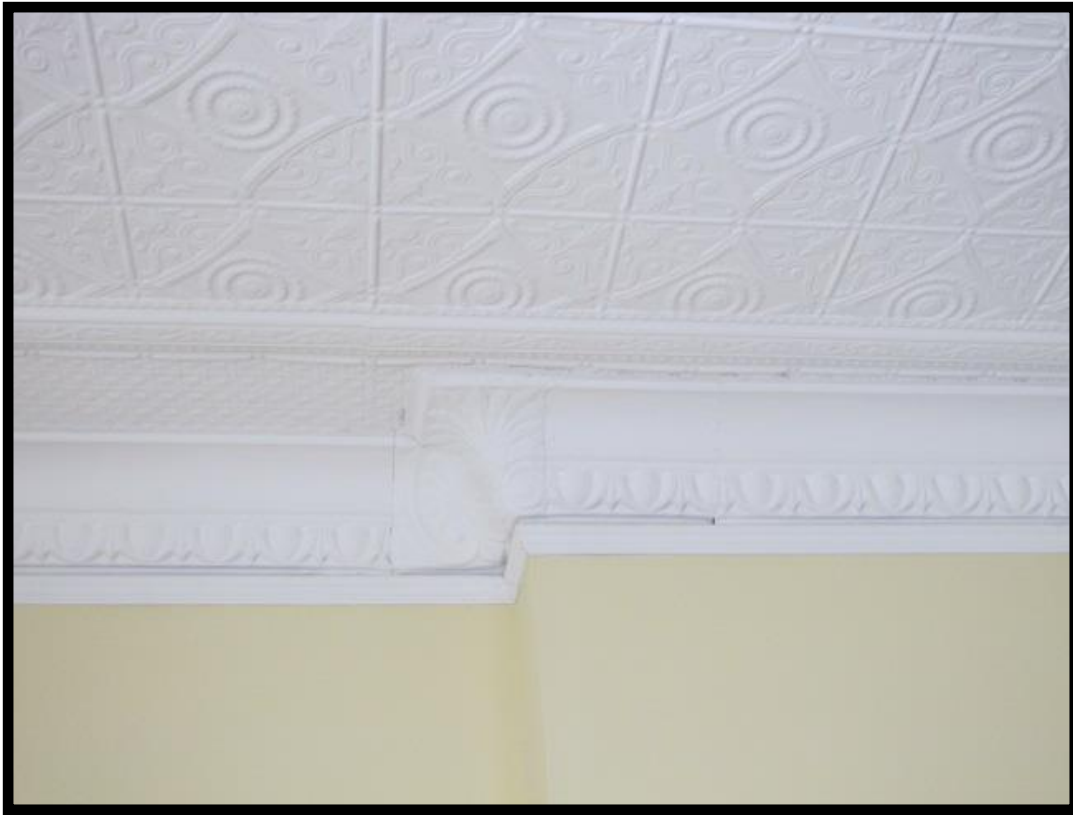
Figure 2.2-15: Ranson House (MK1351), First Floor Ceiling in Southeast Room.
