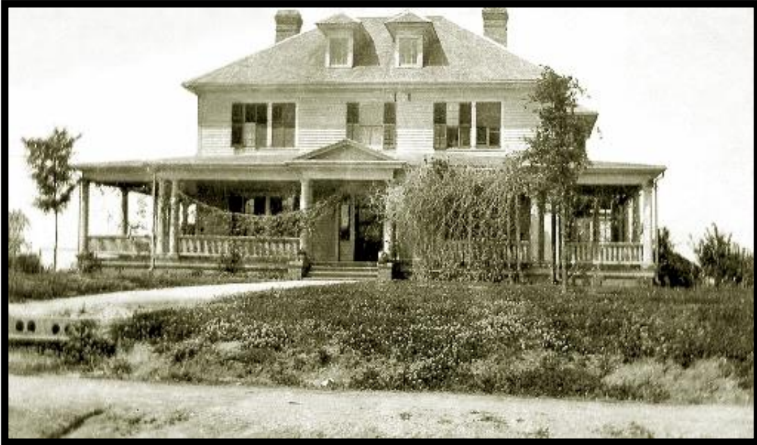
Figure 2.2-28: View of Ranson House (MK1351) Circa 1915, Looking West (Charlotte-Mecklenburg Historic Landmarks Commission 2007a).
