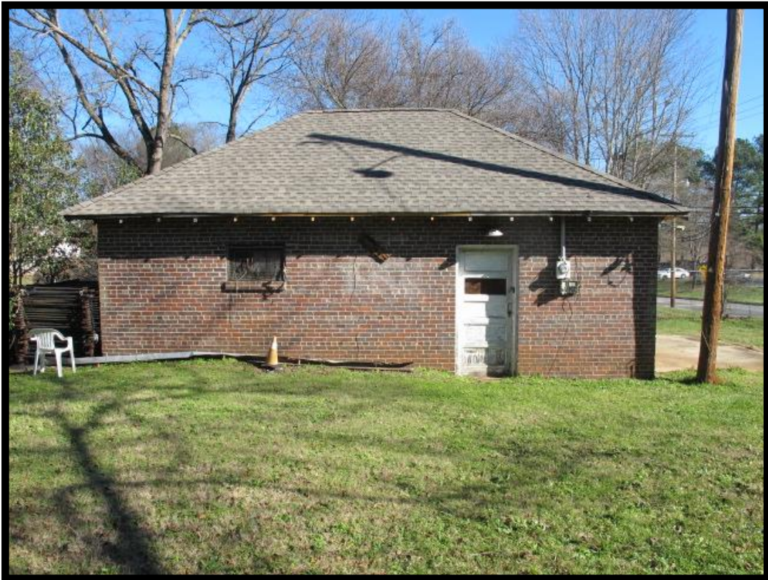
Figure 2.2-32: View of Huntersville Town Jail (MK3299), Looking East.
