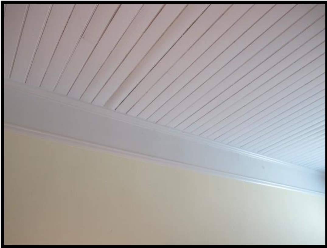
Figure 2.2-17: Ranson House (MK1352), Second Floor Ceiling in Northwest Room.
