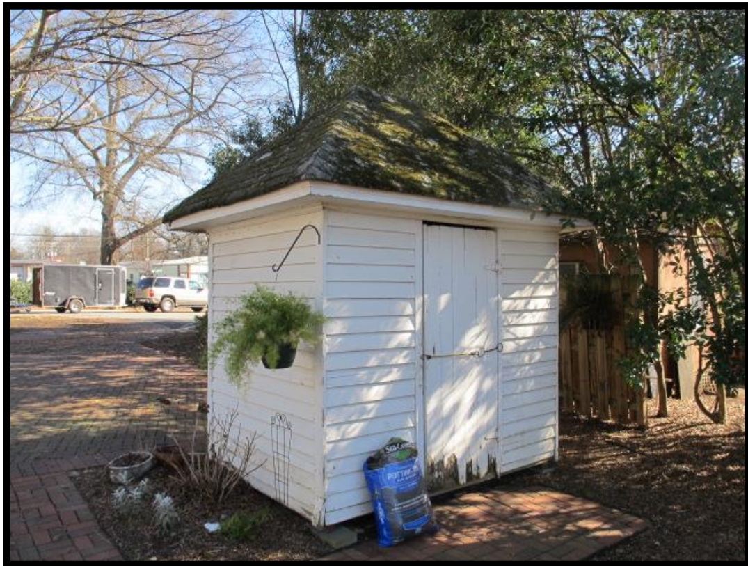
Figure 2.2-22: Ranson House (MK1351), (former) Gashouse Looking Southeast.
