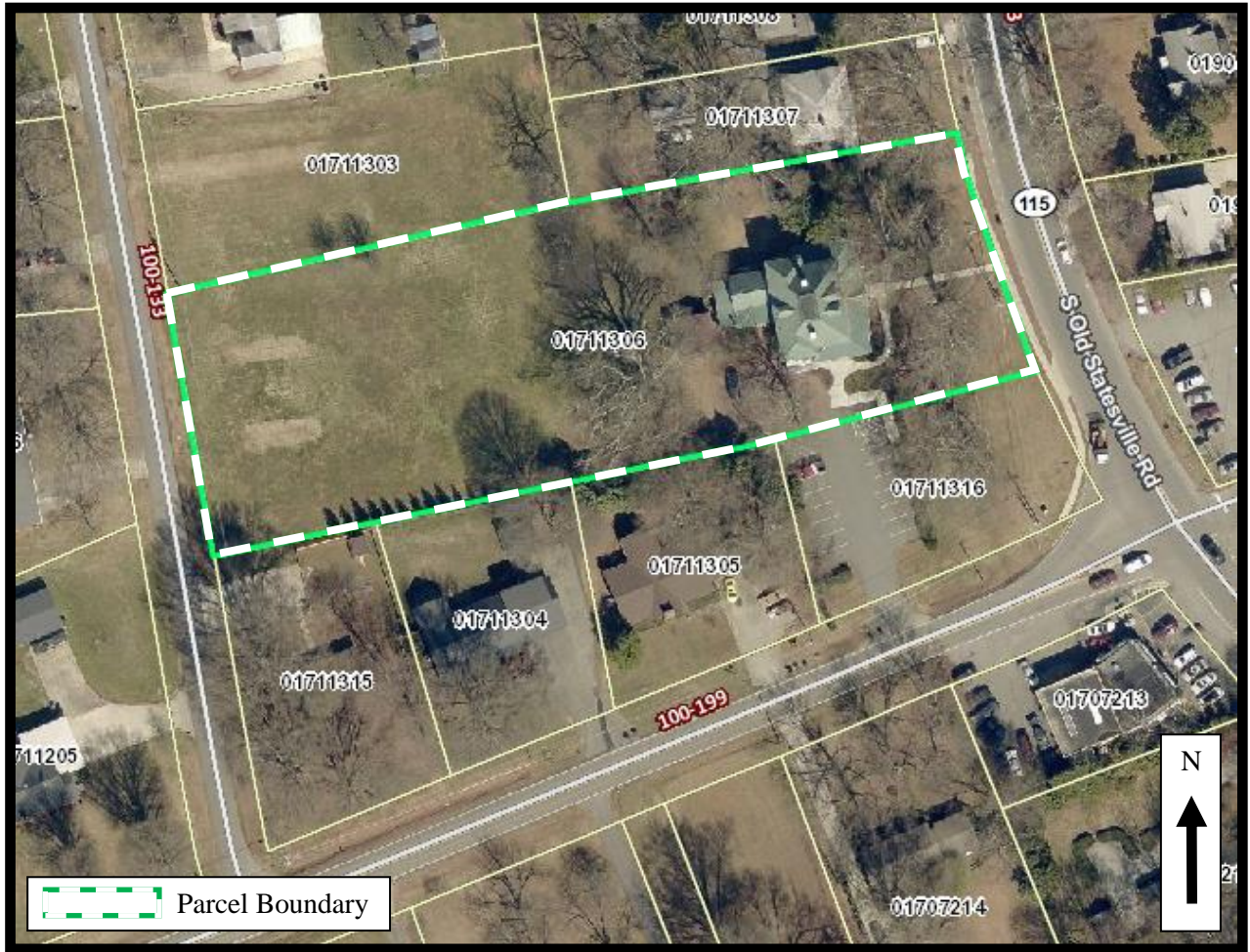
Figure 2.2-30: Aerial View of the Ranson House (MK1351), Showing Proposed NRHP Boundary.
