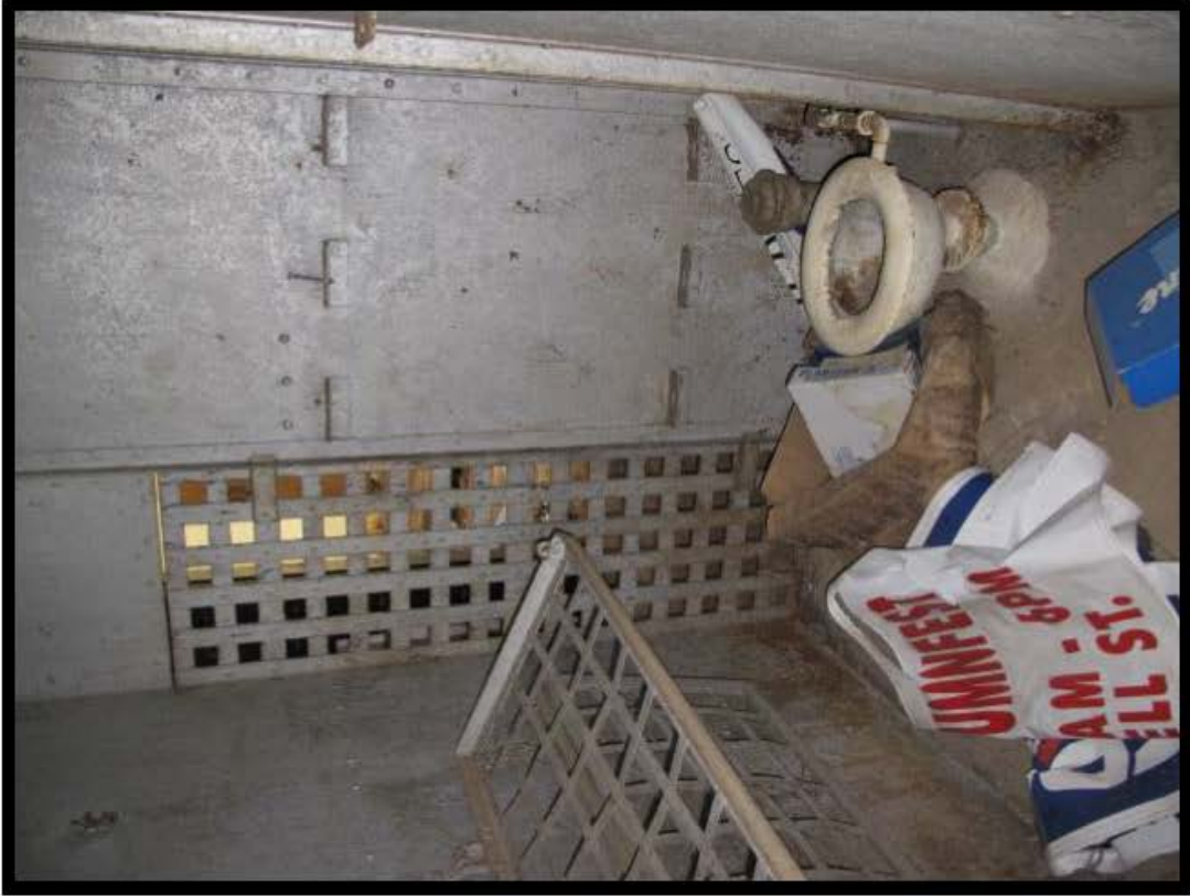
Figure 2.2-38: Huntersville Town Jail (MK3299), View of Smaller of the Two Cells Looking Southeast.
