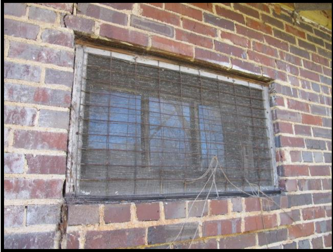
Figure 2.2-33: Huntersville Town Jail (MK3299), Three-Light Hopper Window.
